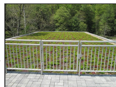
The green roof at Ohio State Park reduces utility costs and filters rainwater
