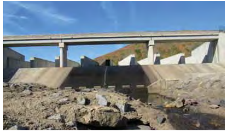
The labyrinth spillway at Lyman Run State Park dam uses a zig-zag design to allow for greater discharge from the dam to prevent dam failure.
