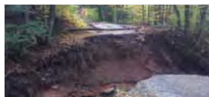
Bridge washed out from flooding.
