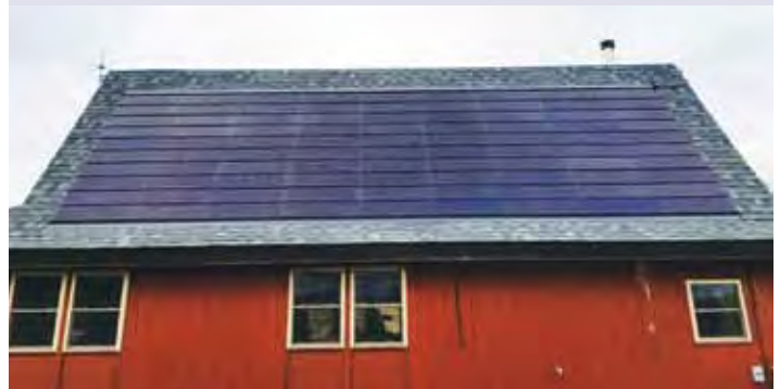
Mt. Pisgah State Park's original solar panels (above) were removed and new solar modules (below) were installed to generate an estimated 6,045 kilowatts of energy per year.
